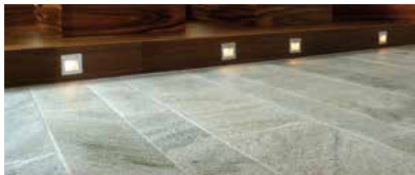
FLOORING LOBBY AND STAIRWELLS RAURISER, granite, green
