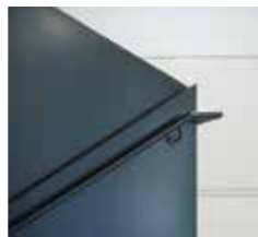
RAILING CONSTRUCTION STAIRWELL Sheet metal construction, color according to architectural concept
