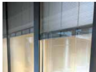
WOOD-ALUMINUM WINDOWS WITH SUN PROTECTION Triple glazing, venetian blinds between the outer two panes of glass, Climawin ventilation and pollen filters in the openable window elements
