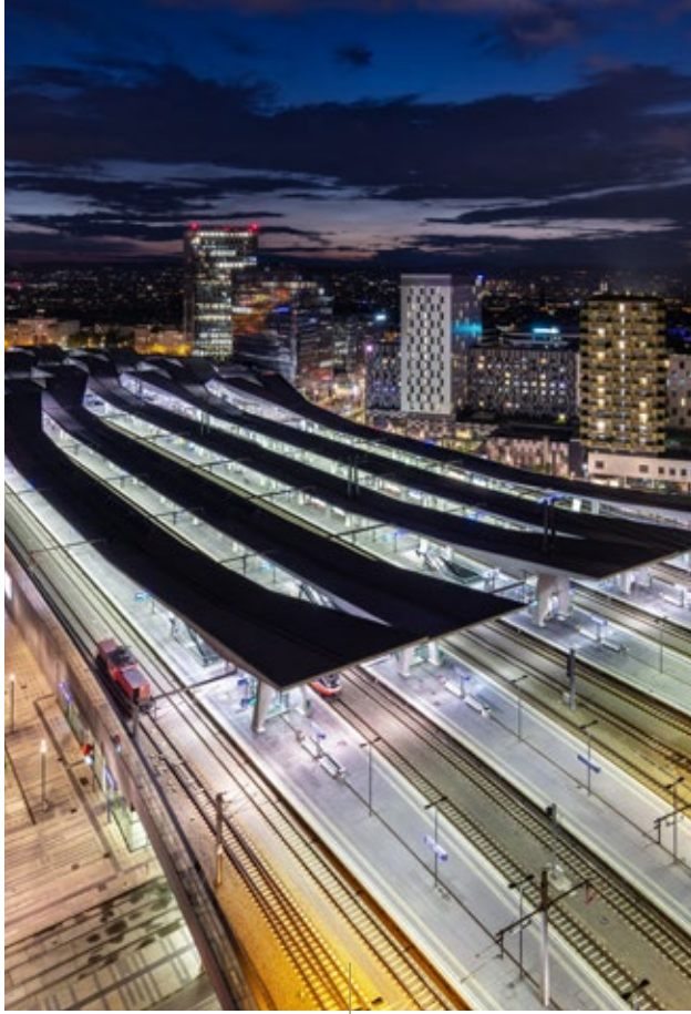
MAIN STATION WITH BAHNHOF CITY
